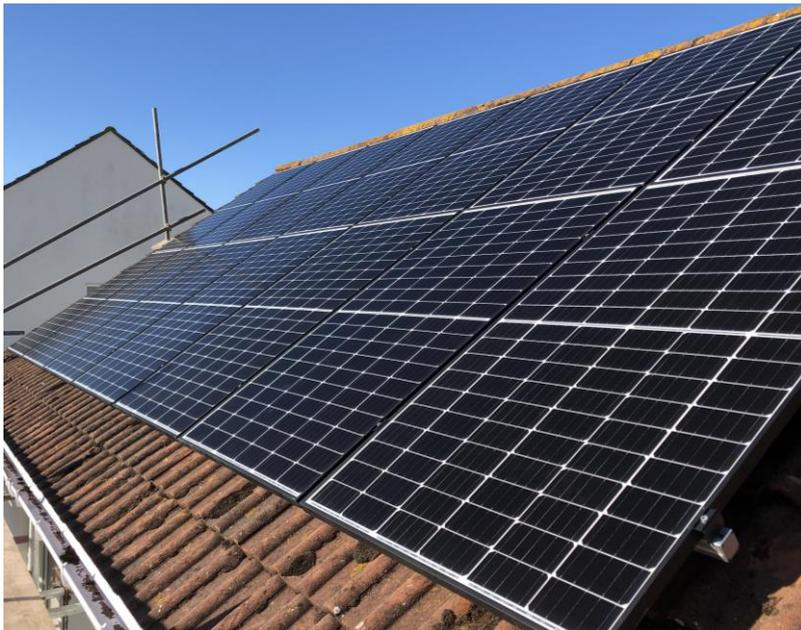
Solar PV uses irradiance from sunlight to create an electric charge in a solar cell. Solar panels are typically collections of 60 of these cells and when connected to other solar panels form a solar array. Electricity produced is fed into a property's electrical distribution board forming a supplementary source of electricity and thereby reduces the amount of electricity that has to be purchased from JE.
