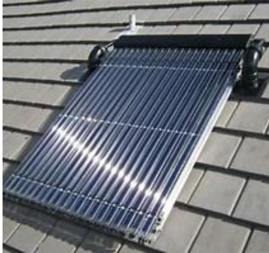
Solar Thermal has been installed by plumbers and heating engineers for many years and uses the heat from the sun to heat water which is passed through extruded tubes on a roof and connects into a property's water system.
